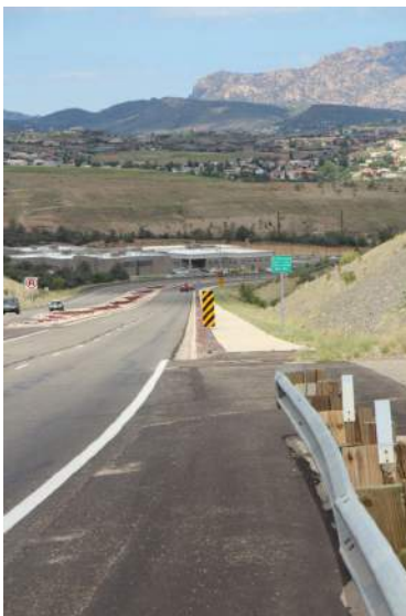
The transition from bike lane to sidewalk on Prescott Lakes Pkwy complicates travel by bike
