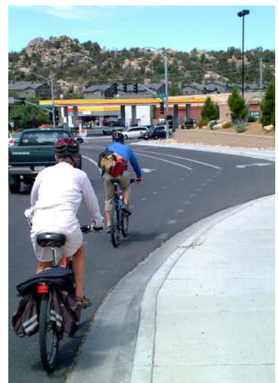
A right turn lane transition at Gail Gardner Way and Iron Springs Road, note the faded paint of the dashed marking for the bike lane.
